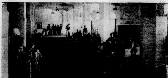
VIEW IN LOBBY OF BARRACKS
