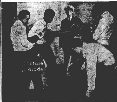
Loading and firing of naval guns is practiced in this loading machine. Dummy shells are used. A job where teamwork counts.
