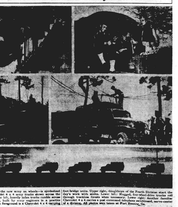
Uncle Sam's motorized force—the new army on wheels—is symbolized by the "down patrol" of Chevrolet 4 x 4 army trucks shown across the top of the photo. Light trucks rumble across a 10-ton-capacity pontoon bridge, built by army engineers in a practice maneuver in 41½ minutes. In the foreground is a Chevrolet 4 x 4 carrying foot-bridge units. Upper right, doughboys of the Fourth Division start the day's work with smiles. Lower left: Rugged, four-wheel-drive trucks roll through trackless forests when necessary. Lower right: Another familiar Chevrolet 4 x 4 carries a port command telephone switchboard, nerve-center of a division. All photos were taken at Fort Benning, Ga.
