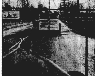
How far ahead can you see? These two station wagons are measuring sight distances, both around curves and over crests of hills. Instruments measure length of restricted sight distances while the crew records the nature of the obstruction.
