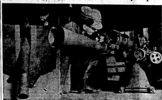
A Finnish gunnery expert is shown examining one of the strange weapons captured from Soviet Russian forces during the recent Russo-Finnish war. The gun, a field piece, is believed to be a device which utilizes explosion gases to produce a forward movement of the gun barrel, thus neutralizing normal recoil. Right: The funnel arrangement is swung aside to show the breech. Experts confess themselves baffled.
