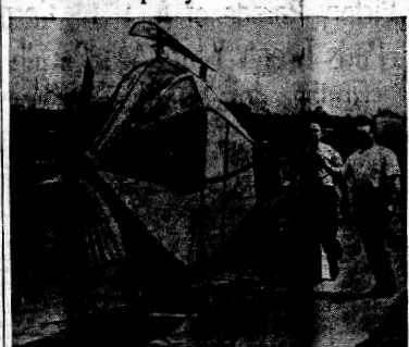
Resembling a winged baby buggy, this peculiar looking contraption is the invention of Paul Foullet (right) of Paris. The propeller is powered by pedals. Mr. Foullet has not yet attempted to take off, but has high hopes that the plane will fly. Ground tests have shown a possible speed of 25 kilometers per hour.
