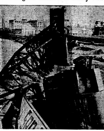
Leaking territorial rains have made this Los Angeles' wettest season in 48 years. The floods underlined and ripped out half of the Santa Fe railroad bridge (shown above) across the Los Angeles river, closing streets and highways with landslides. Hundreds of automobiles were stuck in floodwaters.
