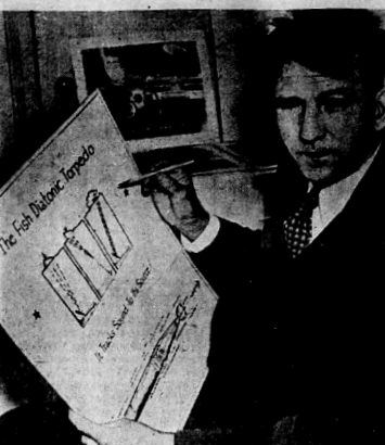
J. Robert Fish, well-known inventor of Springfield, Mass., is shown at his New York hotel with drawings of his "Diatonic torpedo." The sketches show that when used as a mine the torpedo sinks in the bottom and stands upright, at an angle, depending upon currents. Friendly vessels may pass over the mine field safely by using a secret timer.
