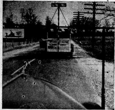
How far ahead can you see? These two station wagons are measuring sight distances, both around curves and over crests of hills. Instruments measure length of restricted sight distances while the crew records the nature of the obstruction.
