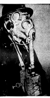
Smoke-filled interiors held no fear for fire ladies equipped with this combination gas mask and telephone. The mask protects the fireman as he "phones" directions for fighting a stubborn blaze.
