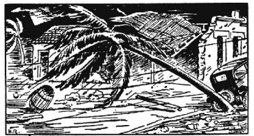
Roofs Went Flying Off Houses.
