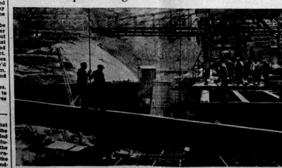
Swinging a steel beam into place to close the last gap in one of the most unique bridges ever built. Three thousand feet long, one hundred seventy-five feet high, this half-million dollar structure will be swallowed in six months by the rising concrete of Grand Coulee dam, being built by the bureau of reclamation on the Columbia river in Washington. The bridge was constructed as the most economical means of moving concrete from two great mixing plants, one at either side of the river, over the foundation area of the dam, 368 feet wide by 3,000 feet long. A part of the west section of the dam can be seen in the background.
