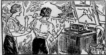
A Tottering Wall Fell With a Crash.
