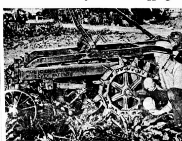
Of almost human ability at "topping" and digging sugar beets is the recent invention of John Devey, Jr., of Glendale, Calif., shown here with his device. Weighing 3,000 pounds, the machine in one operation slices the tops from the beets, and digs them from the ground 6 times as fast as the average worker.
