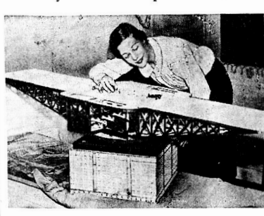
A model of a rotary elevated airport, designed by Captain Charles Frobisher was exhibited at the Inventions Exposition held recently in Central hall, London, England. One of the big advantages claimed for the rotary airport is that it can be turned in the direction the wind is blowing, thus facilitating the take-off and landing of planes.
