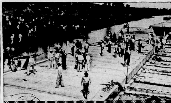
Vast public works allotments for work on the Mississippi river have put thousands of men back to work. This photograph shows workmen, under the direction of army engineers, fabricating concrete mattresses at Profit Island, La.
