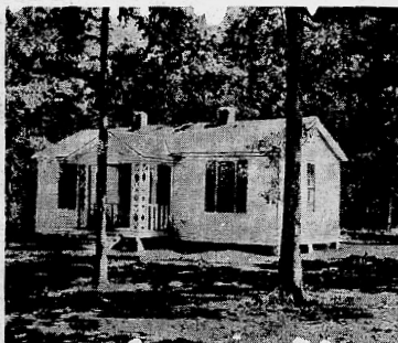
One of the model homes built in Model-shed county, Arkansas, in a project for which $12,000,000 of government funds has been allocated and a tract of 16,000 acres of cut-over land bought at $2.50 an acre. The houses have been built at an average cost of $1,100 each.
