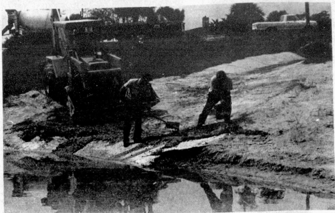
Lake Verona— ONCE AGAIN CITY Employees made repairs to storm sewer spillways on Lake Verona after a small shower last week from the left: Eldon Sizemore and Willis.
