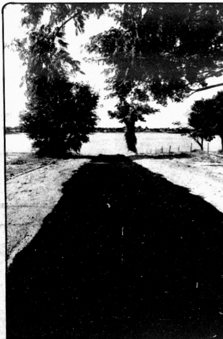
THIS DRAINAGE DITCH at Lake Isia has prompted charges that it is polluting the lake and endangering the quality of one of the city's better lakes. Councilmen
