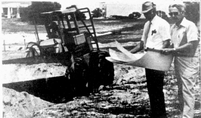
DR. WILLIAM STALLARD, President of South Florida Junior College and architect Robert B. Murphy check over blueprints as a front end loader removes
