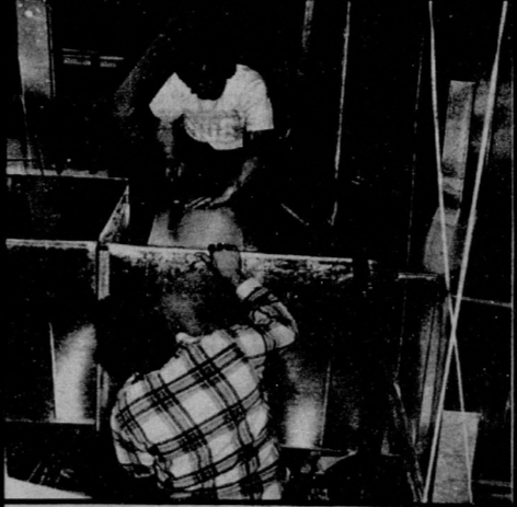
Larry McKinney and Don Roth trim excess duct for a proper fit to help make Long's Carrier Air Conditioning efficient and worry free.
