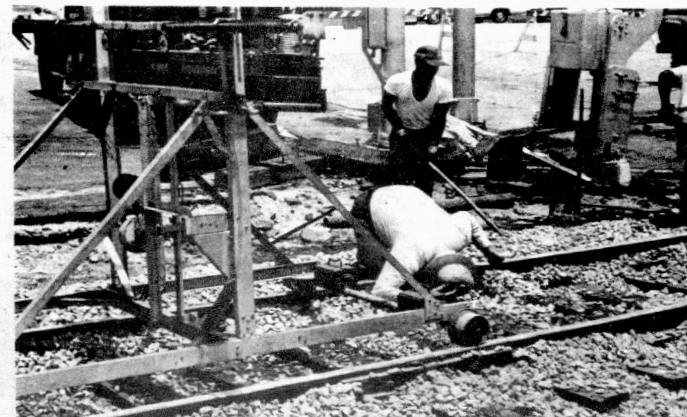
Howard checks to make sure everything is o.k. after new ties and rock have been replaced before the machine aligns the track.
