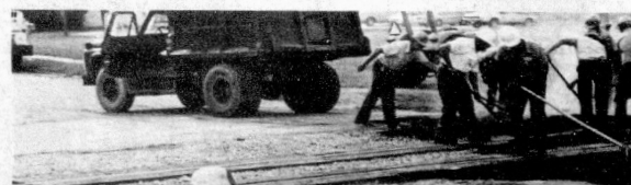
Howard checks to make sure everything is o.k. after new ties and rock have been replaced before the machine aligns the track.
