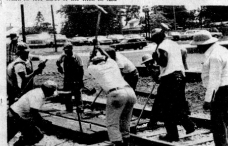
Some of the hard labor still has to be accomplished by hand as is shown in the photo above.
