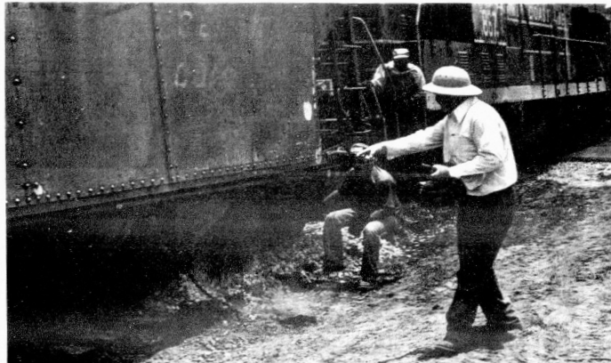
Milton gives instructions to one of his crewman while new rock is being placed on the bed of the railroad track.
