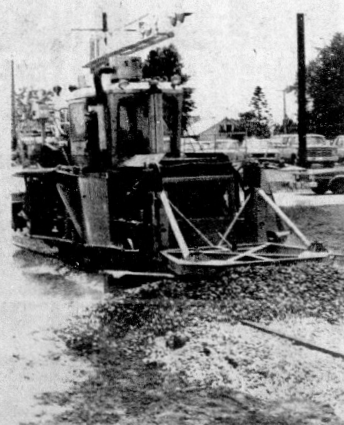
The rock spreader helps make the maintenance crews job a little easier.
