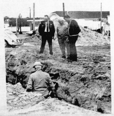
Footers for the new fire station on Pine Street and Delaney Avenue. Sunphoto by Lew Miller.
