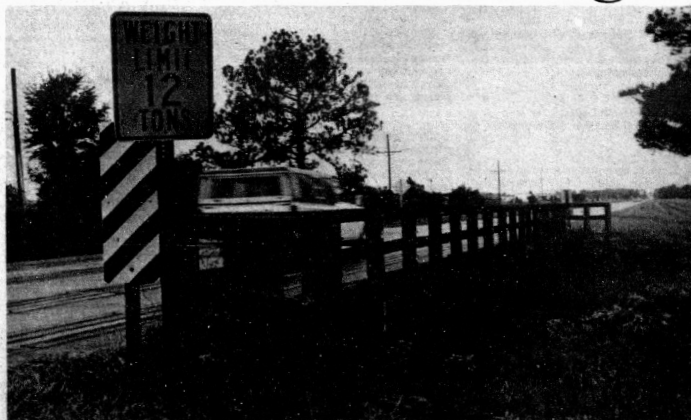
This wooden bridge over Bonnet Creek will soon be replaced.
