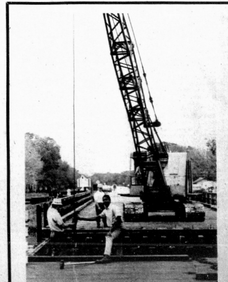
POLK COUNTY ROAD crews are hard at work constructing this new span linking Avon Park with the Avon Park Bombing Range and the state correctional institution and hope to have the project finished sometime next month.
