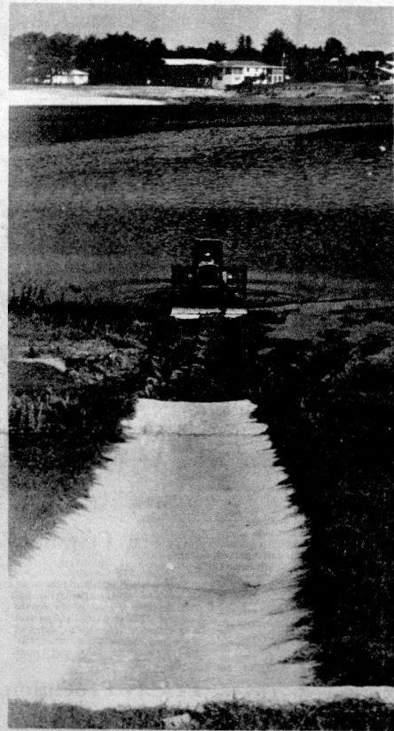
CITY WORKER, JACK Elder, starts another pass in shoving sand up to the end of a street runoff spillway on Lake
