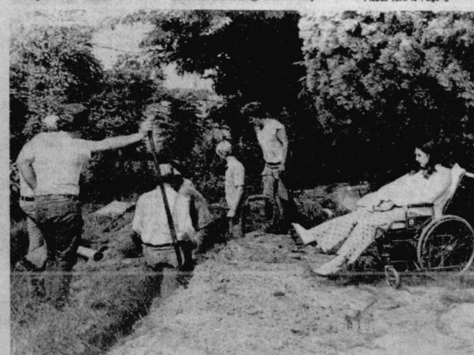
AS ONE OF their projects the newly organized forces of Avon Park installed and connected a sewer line to the
