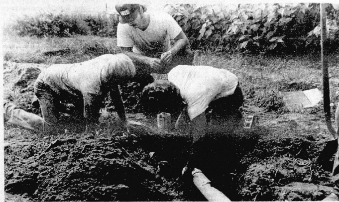
JAYCEES MAKE a connection as the group installed the sewerline from the Johnson house plumbing to the city sewer line. From the left: Joe Murphy, Foy Hall and Guy Nealis. Sunphoto by Lew Miller.
