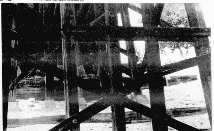
THE 56 some year old wooden humpbacked Palmetto Street bridge across the Seaboard Coastline Railroad tracks will be getting a new lease on life, as timbers for repairs have been unloaded at the Pleasant St. trestlehouse.
