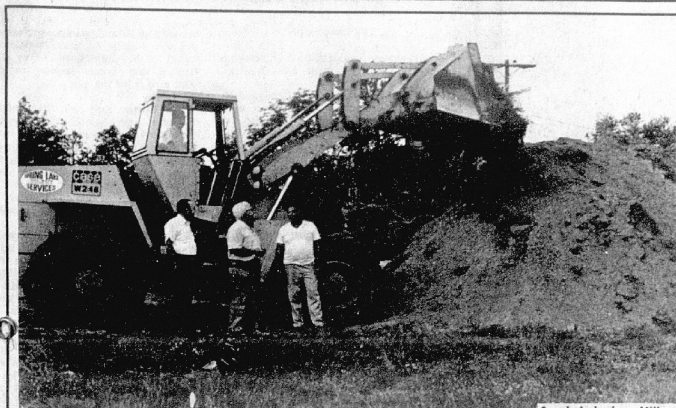
INSTEAD OF THE usual shovel, a front end loader was used for ground breaking for the new Avon Park Fire Station on Delaney Ave. and Pine Street. From left: Driver Ronnie Brock, Mack general superintendent for Wayne Flowers, Fire Chief; James "Jim" Blackwell and Co., Inc. Contractor.
