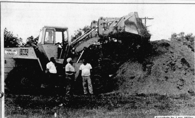
INSTEAD OF THE usual shovel, a front end loader was used for ground breaking for the new Avon Park Fire Station on
