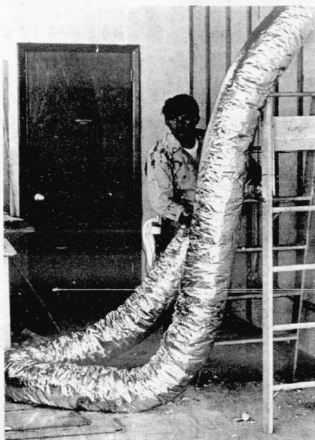
THE PAST FEW weeks have been hectic at the Avon Park Sun, as our offices are undergoing a complete remodeling.
