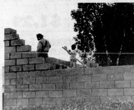
SATURDAY WORKMEN FINISHED laying the block walls of the addition to the Avon Park Library, which will house
