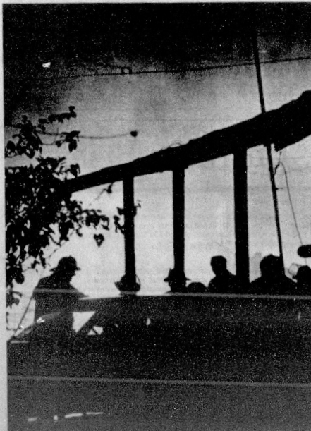
FIRE DEPARTMENT TRAINING officer Capt. Allan Ball using diesel fuel saturated the inside of an old house in
