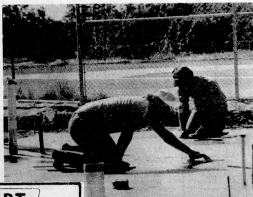
WITH HIS NAME inadvertently left out of last week's outline, Gerald Cooper (left) was reported as the prime mover in the pouring and finishing of the floor of the concession stand-press box building at the Ball Park Complex. Joe Jackson keeps pace at the right. Sunphoto by Lew Miller.
