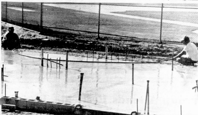
AFTER ALMOST A year of talking the floor of the field building was poured last Saturday at the baseball complex (near the airport). Steve Walker (left) and Joe
