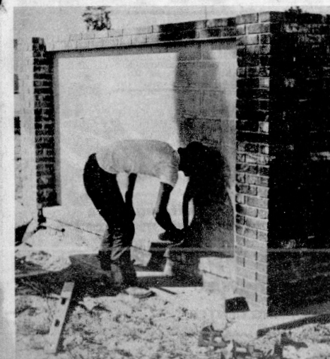
CLEANING UP, Wayne McCall, Avon Park, a five year member of the Florida National Guard gets ready to apply the finishing touches on the masonry sign for
