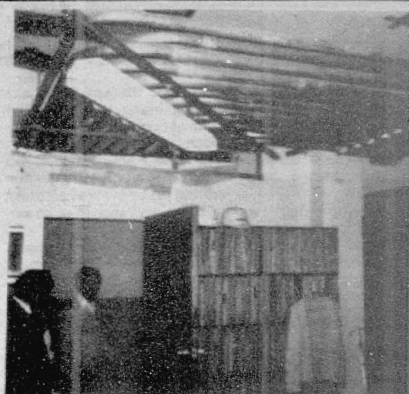
PLANT CITY HOSPITAL HAROLD RICHARDSON, DAVID "SCOTTY" GARDNER LOOKING OVER JOB
