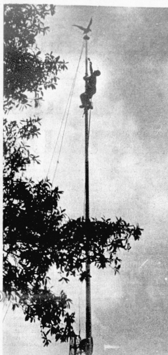
George Johnson Applies A Quick Coat Of Paint To The Flagpole On The Mall
