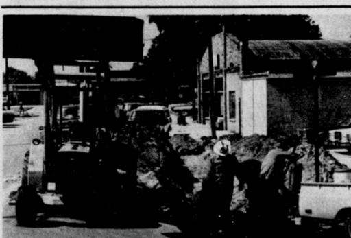
CITY EMPLOYEES ARE preparing to cut off the bell end of a clay sewer pipe to complete the two lines from a catch basin in front of the Ford place. The intake end of the old line was too high while a second line crossing
