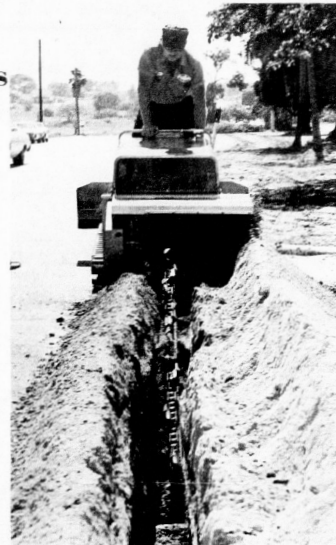
THE CITY'S NEW trencher gets its first workout as Joe Willis, at the controls, watches it dig through street paving for an irrigation line on the Mall. Photo — Miller
