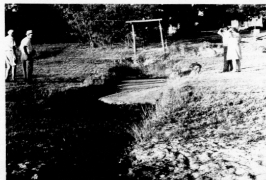
Raw Sewerage Cut Channel To Lake
