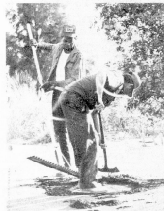
FIRST IT'S COVERED, then you uncover it. Superintendent of Jones Contracting, Dean Warner, with shovel, Matlack, Fla. and Lee Freeman, Ft. Myers, uncovered the manhole and grade the hot mix around it as the street was being paved. Sunphoto — Miller.
