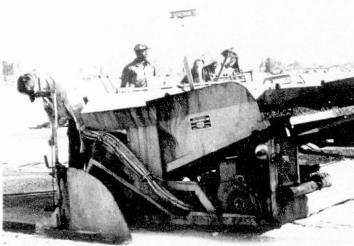
WITH LAKE BOULEVARD paving completed workmen of Jones Contracting, Ft. Myers, were getting ready to complete W. Edgewood St., last Thursday. Making depth
