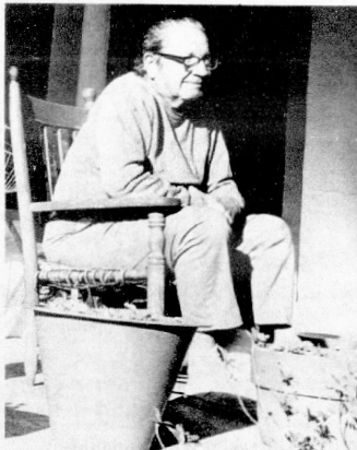
FRONT PORCH SUPERINTENDENT Carl Horning on S. Park Ave. watches the street paving at the side of his house and stated he would be glad when it was finished. To get rid of the dust and rough streets. As to looking on the sewer line he would like to see the sewer plant working good first. Sunphoto - Miller.
