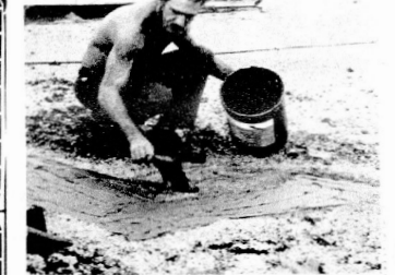
"IF IT'S WORTH doing it's worth doing right the first time" is the philosophy of Ray Marshall of Sebring as he repaired a leaking patched area on the roof of the Avon Park High School last Saturday afternoon. His helper was Dave Moody of Lake Placid. Photo: Miller.
