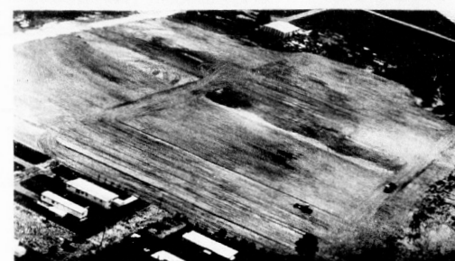
THE ROAD GRADER and earth mover working on the Ball Park Complex appear small in relation to the 20 acre ball park. The park will have a little league field, a senior
