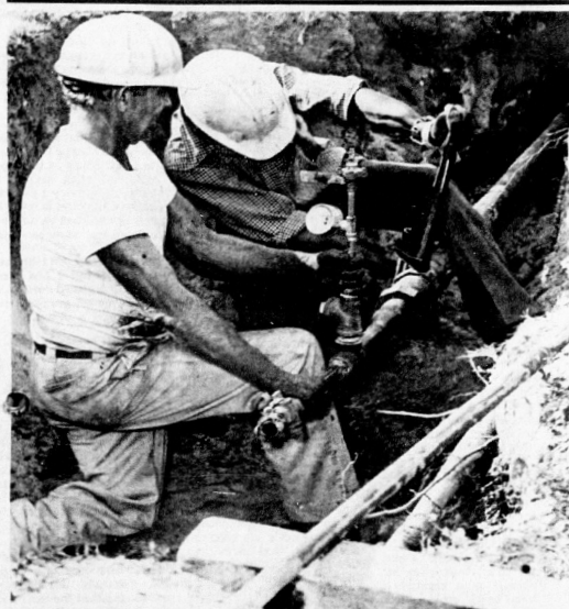
MUSCLE POWER GETS the job done as Thurman Toffen steadies the special fitting and Reggie Graves, (both of Longwood) applies pressure with a pipe wrench to remove the fitting after blowing sand from a pipe driven under W. Main St. by the J and S Underground Utilities for an extension of the Florida Gas lines. Photo—Miller.
