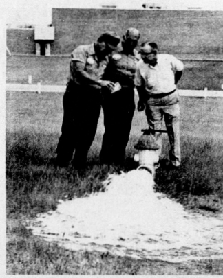
HIGH SCHOOL CUSTODIAN VINYL STILL leans over to see how much sediment was being flushed out of the city water mains by Paul Backman and Joe Willis (right), following the addition of chlorine to the water supply. Photo—Miller.
