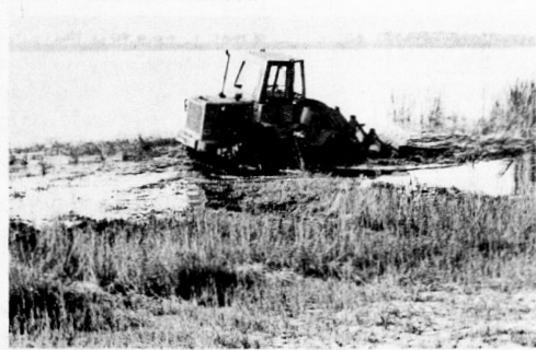
THE GRASSY WATER covered second shore line of Lake Letta makes a smooth working surface for Emmitt Richards as he leads the yard and a half bucket of the Highlands County's articulate end loader with sand and grass last Friday. A channel had to be cut through the washed in second
