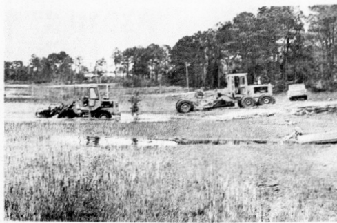
THE PUBLIC BOAT launching ramp on South Lake Letta gets a cleaning out as Roy Bennett Highlands County Maintenance Supervisor for this area brought his crew and equipment to make it easier for boaters to
