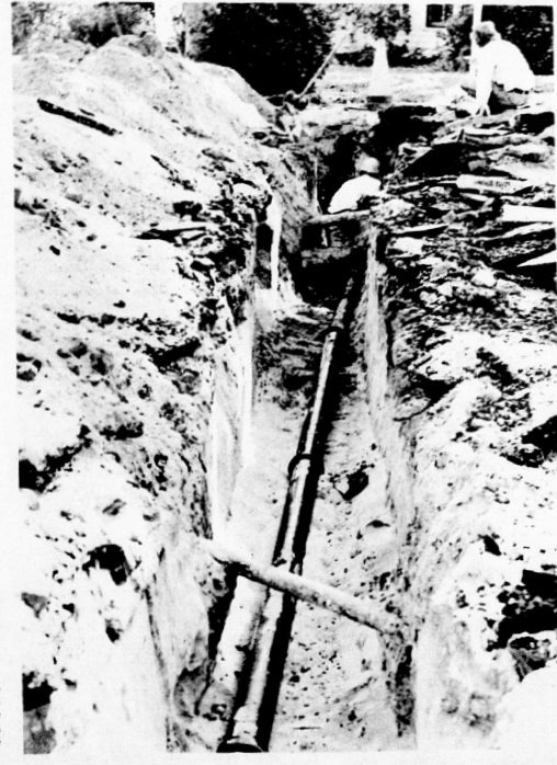
DOWN IN THE earth under other pipe lines and stopping the Lake Avenue traffic goes this sewer line from the new telephone switching center as workmen are tapping into a sewer junction box to make the necessary connection to complete the hookup.
