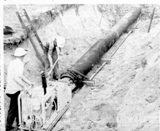
STAR TELL, INC., sub-contractor to sub-contractor McCollum Industries specializes in driving steel pipe under roadways for sewer lines, water and other utility lines. This section of a 16 inch steel pipe 110 feet
