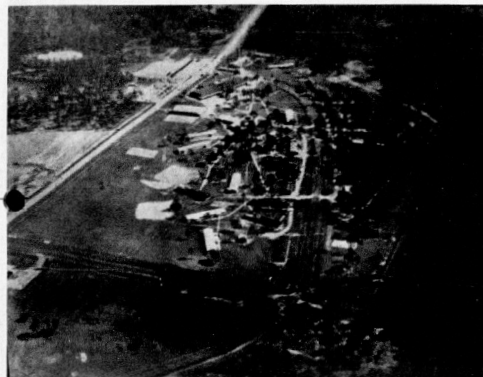
AERIAL VIEW OF the Avon Park Correctional Institution.
