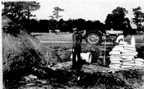
SITE WORK CONTINUES at the location of the new APCI kitchen-dining room facility with Charter Builders superintendent Don Loftis checking work progress along the road adjacent to the building site. In the
