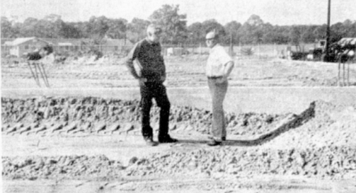
NEW APCI FACILITY. With the concrete foundation in, building of the new kitchen-dining room facility at APCI in well underway. The 8,000 square foot complex was originally slated to cost $500,000 but the state has requested a change order eliminating the air conditioning which is under discussion with the contractor and
