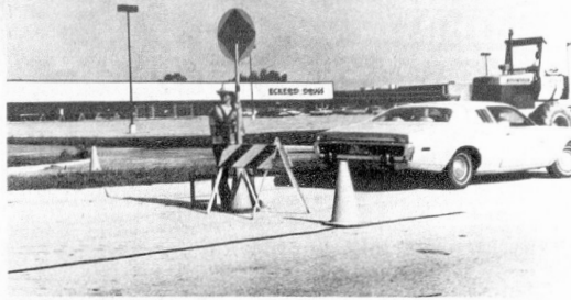
WOMEN JOIN MEN in working on highway repairs as Laurie Simpson of Lakeland signals approaching traffic to slow down for work on the traffic storage lane at the
