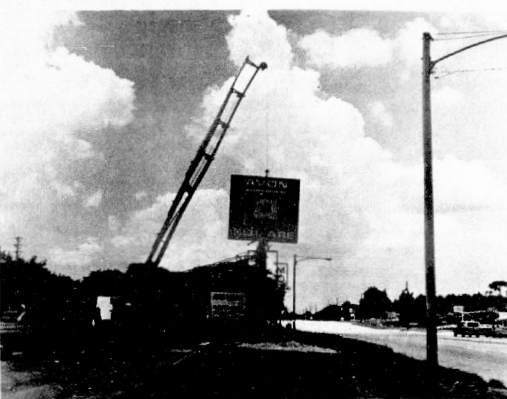
THE AVON SQUARE Shopping Center sign was placed in position Monday to take the place of the temporary sign that was erected when construction started at the complex.
