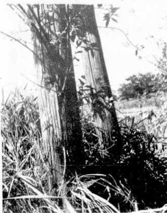
BRUSH SEED GERMINATED in the damp wood of this irrigation intake pipe support post with the roots coming to the surface of the post and growing into the soil two feet below. Photo—Miller.
