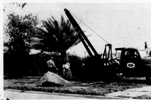
EMPLOYEE D. L. Jackson directs a truck driver Bill Revels in transplanting a palm tree that was moved from Michigan Ave. will be constructed across the Mall west of the railroad tracks. Photo—Miller.
